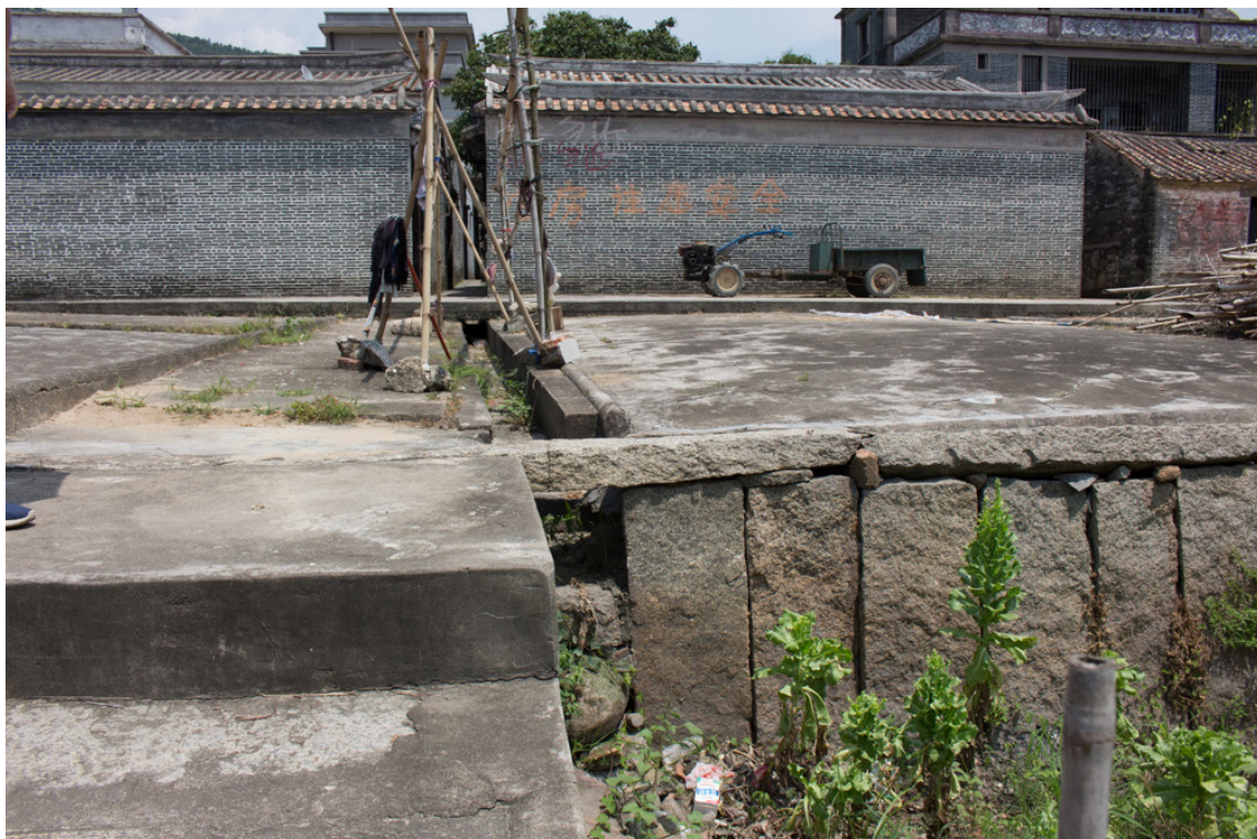
Figure 4. Drainage system parallel to the lanes, collecting water in the pond. Majianglong village, Kaiping County (source: photo by the author, May 2018).
